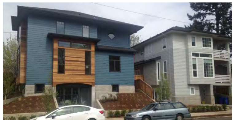
Wider eaves help to reduce the perceived scale of a house. Bay window projections also help to break up the massing of building walls.
